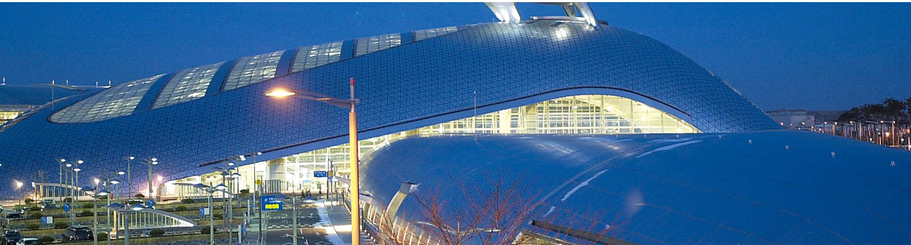
Incheon International Airport
