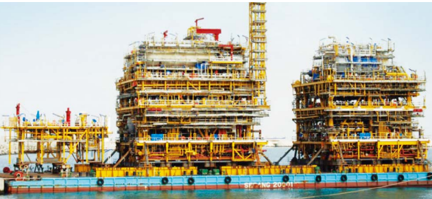
FPSO top-side modules
